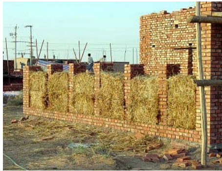
Figure 1.4 Inner Mongolia, China. Workers stacking bale walls (Lerner, K)
