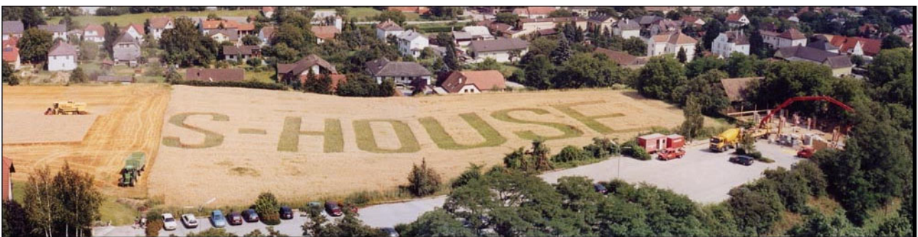
Figure 1 The S-House in Böheimkirchen / Austria is made of renewable resources. The logo growing in a corn field. © GrAT
