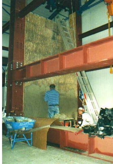
Figure 5: Render application over mesh for two-storey wall. (Photograph P. Florence)
