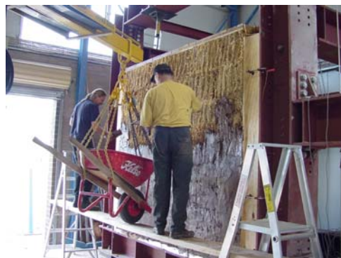
Figure 6: Earth render application. (Photograph P. Florence)
