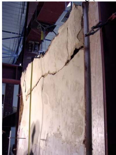
Figure 15: Earth rendered wall after test, note cracking (Photograph S.Overmeyer)
