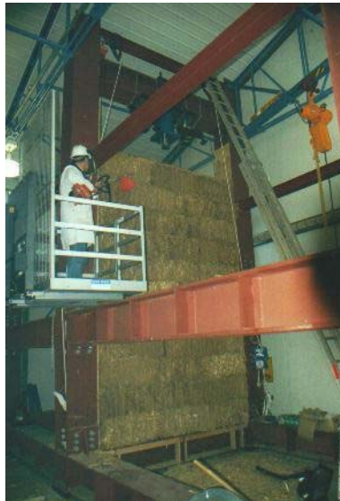
Figure 4: Trimming two-storey bale wall to size. (Photograph P. Florence)
